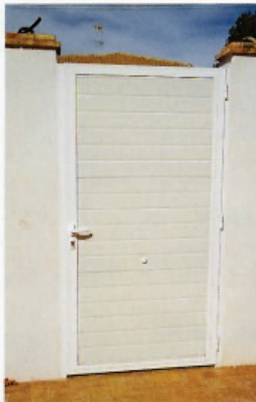
Puerta peatonal, vista interior
